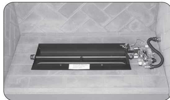
Fig. 17-2 Center burner in fireplace
